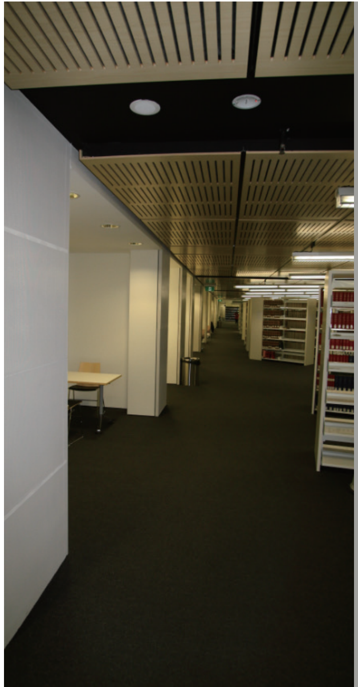
Figure 7 Full-height displacement outlet integrated in column
