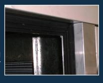
**Door Seal** Mechanically fixed rubber door seal cover full flange.
