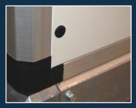
Panel Fixing Panels screw fixed within nylon inserts and caps. Protective film to be removed on site.
