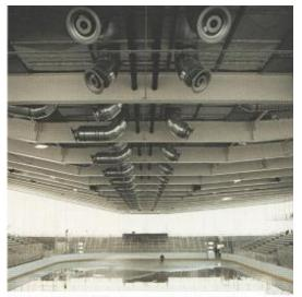
extremely quiet operation of less than PNC30. In contrast, similar 16 m high air distribution at the Christchurch Sport & Entertainment Centre has a noise level of about PNC35 due to the higher discharge velocities required for effective heating; additionally, 50% of the return air is drawn from a low level to aide heating performance.
